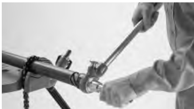
Figure 2 – Reaming End of Pipe
