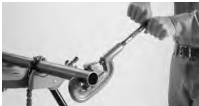
Figure 1 – Cutting End of Pipe
