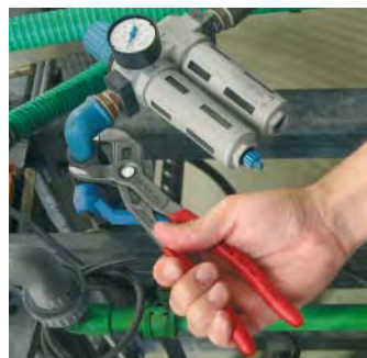
Operation on pneumatic pipes
